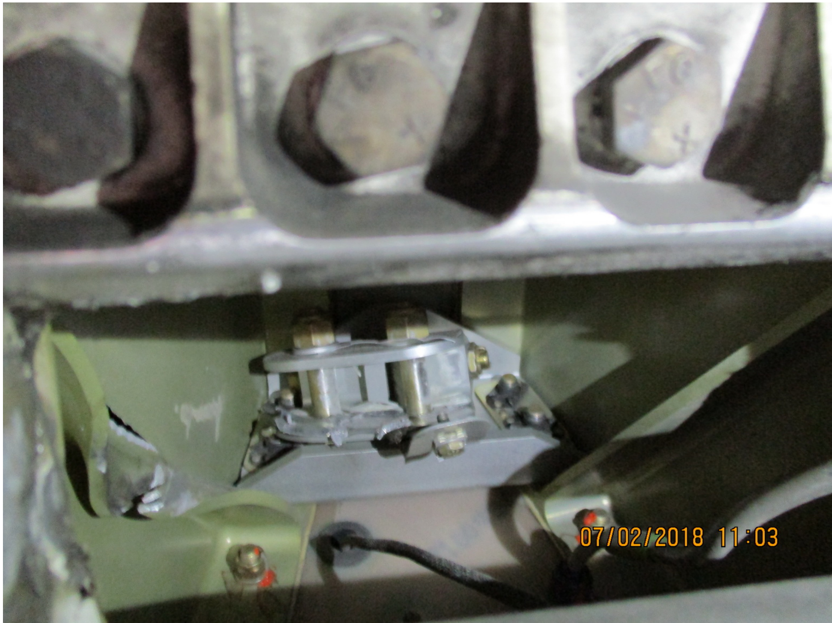
Photo 1 – View of damage to the forward wing spar (Courtesy of FAA)
