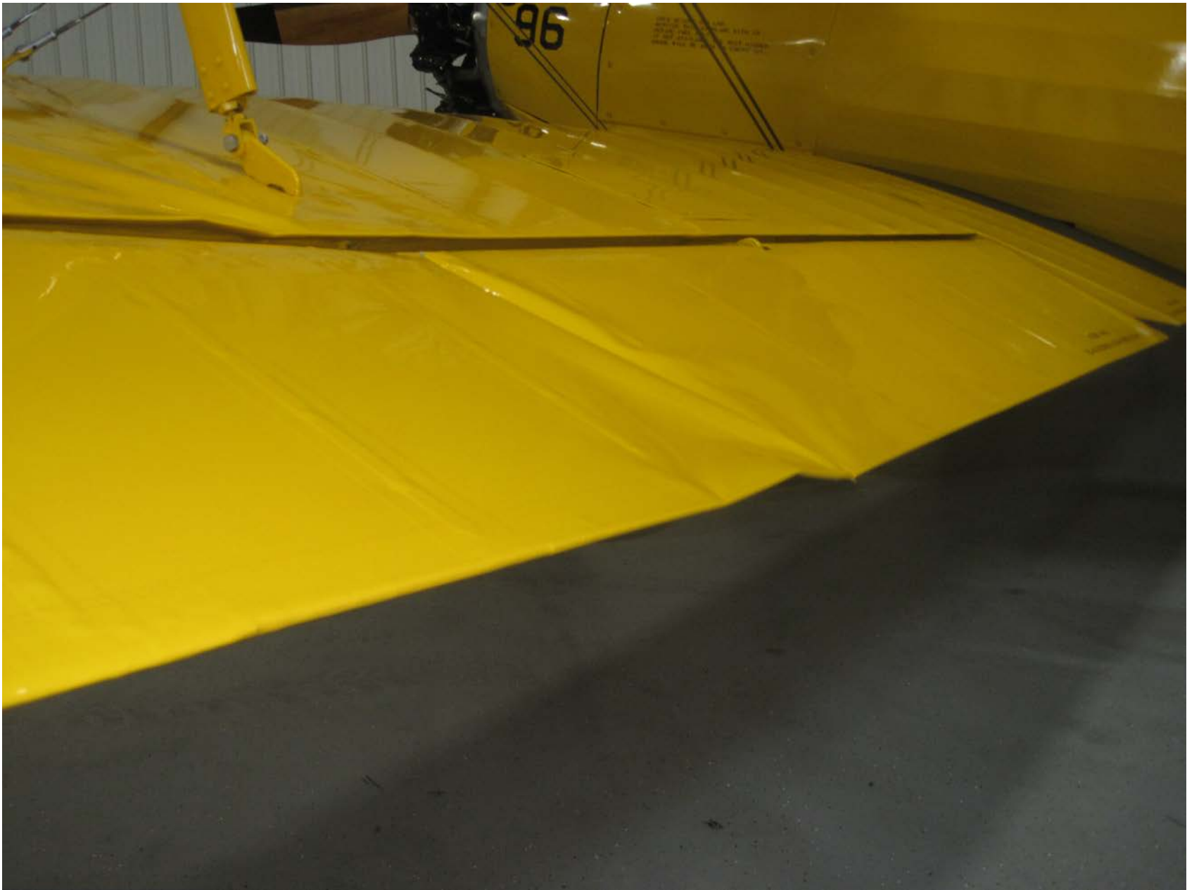
Photo – View of damaged left wing (Courtesy of the FAA)
