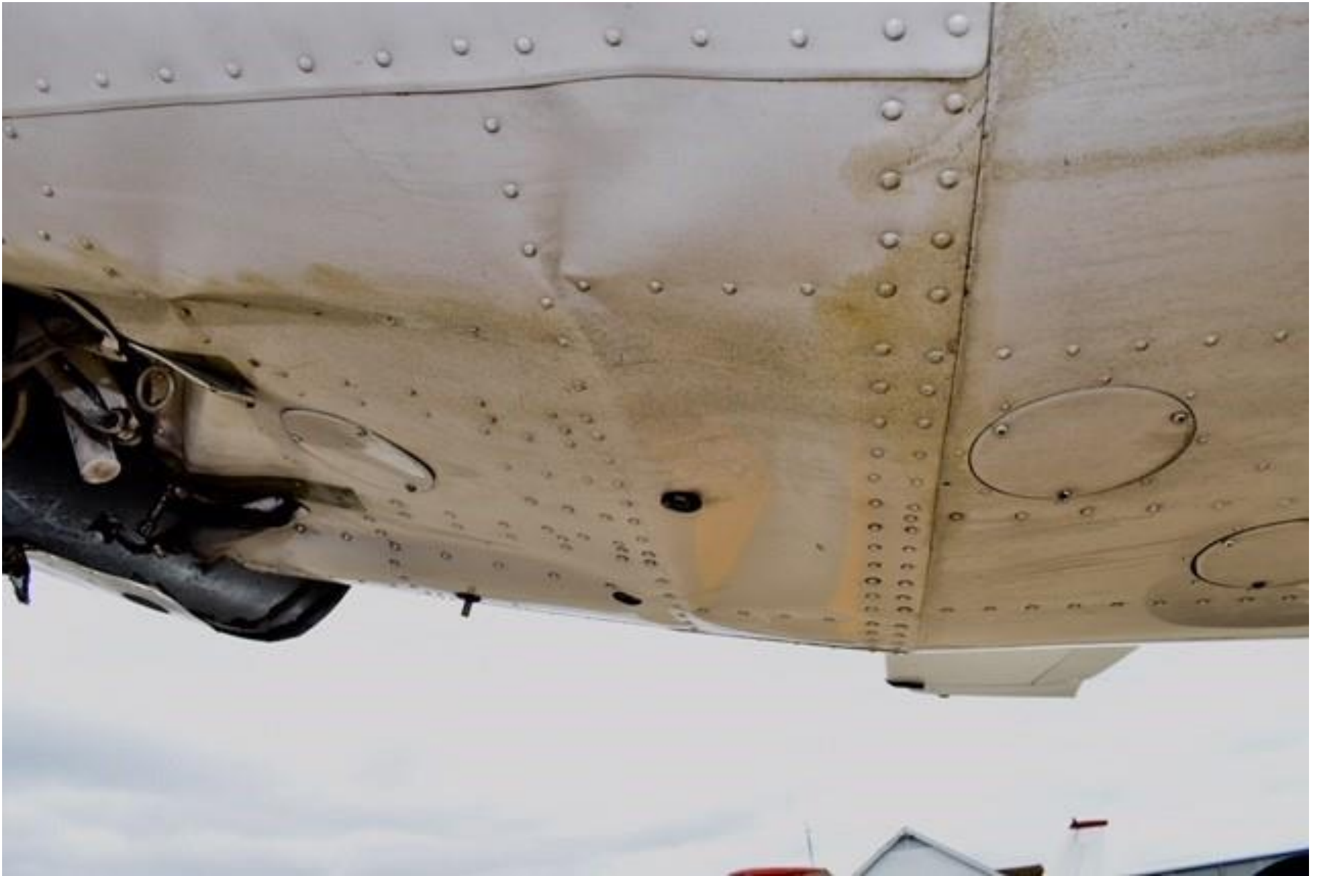
Photo 1 – View of damaged lower forward fuselage (Photo courtesy of the flight school)
