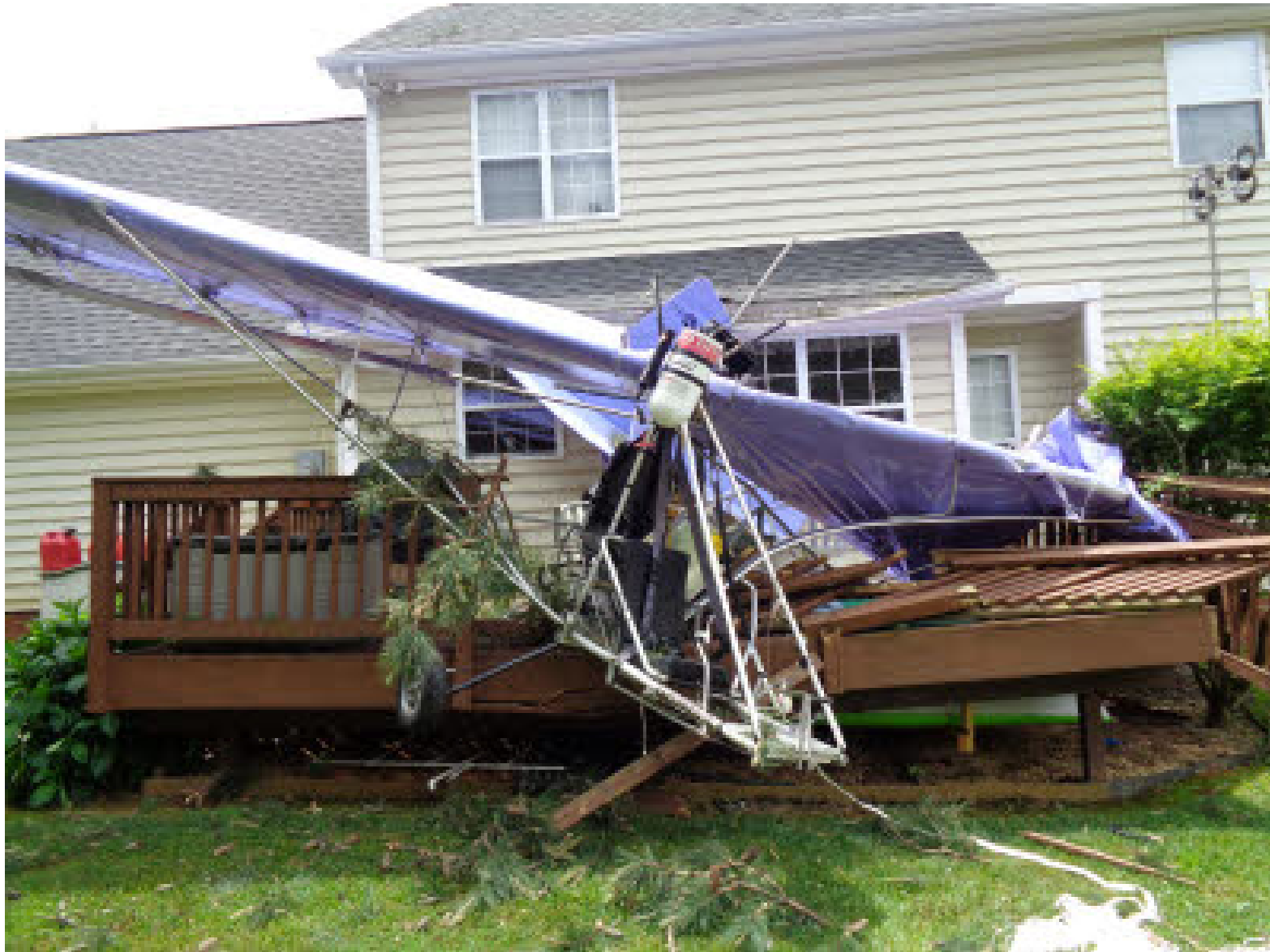
Photo 2 – View of airplane on residential house deck from front (Photo courtesy of the FAA)
