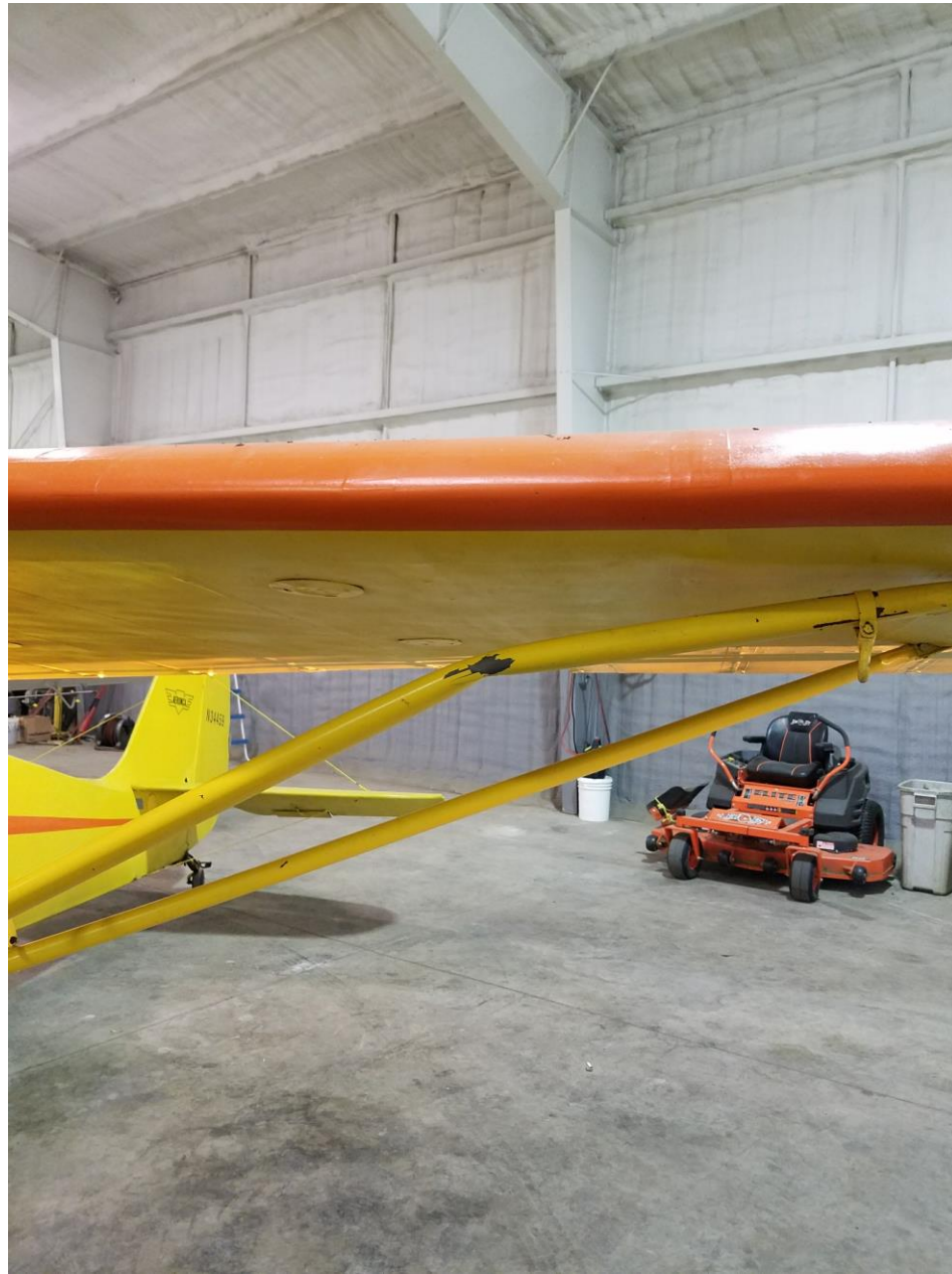
Photo 1 – View of damaged left wing lift strut (Photo courtesy of the owner)
