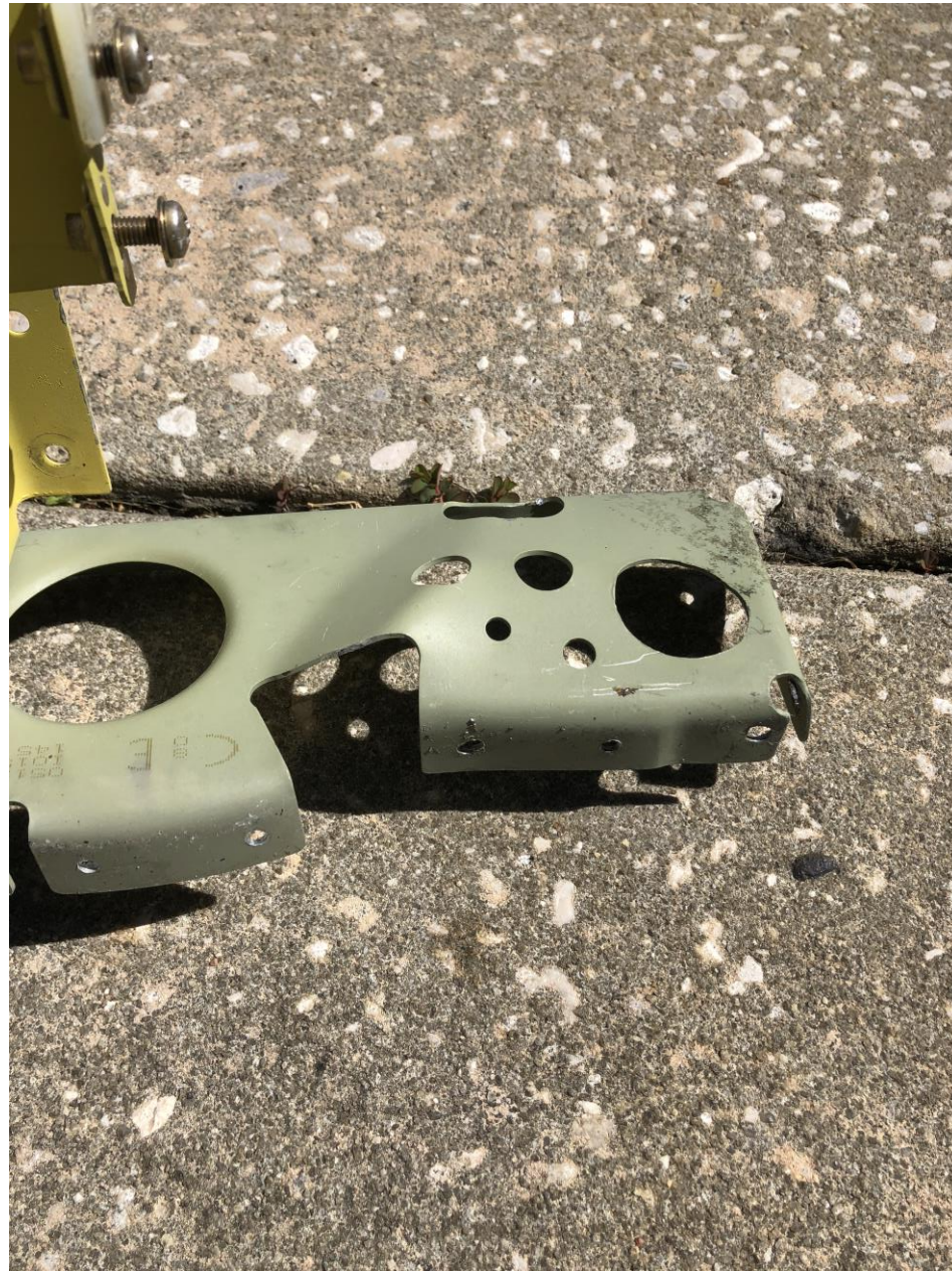
Photo 1 – View of removed floor rib (Photo courtesy of the operator)
