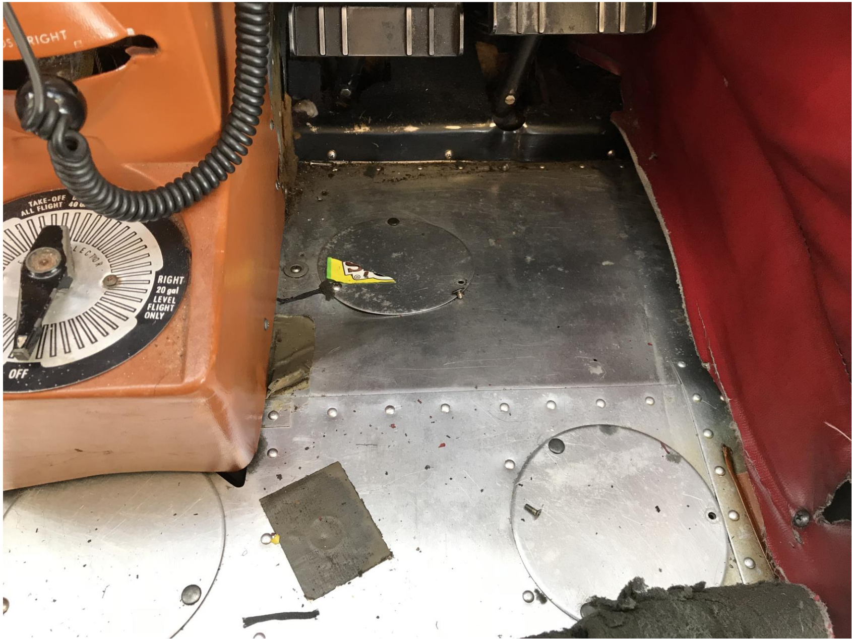
Photo 1 – View of damaged floorboard (Photo courtesy of the FAA)
