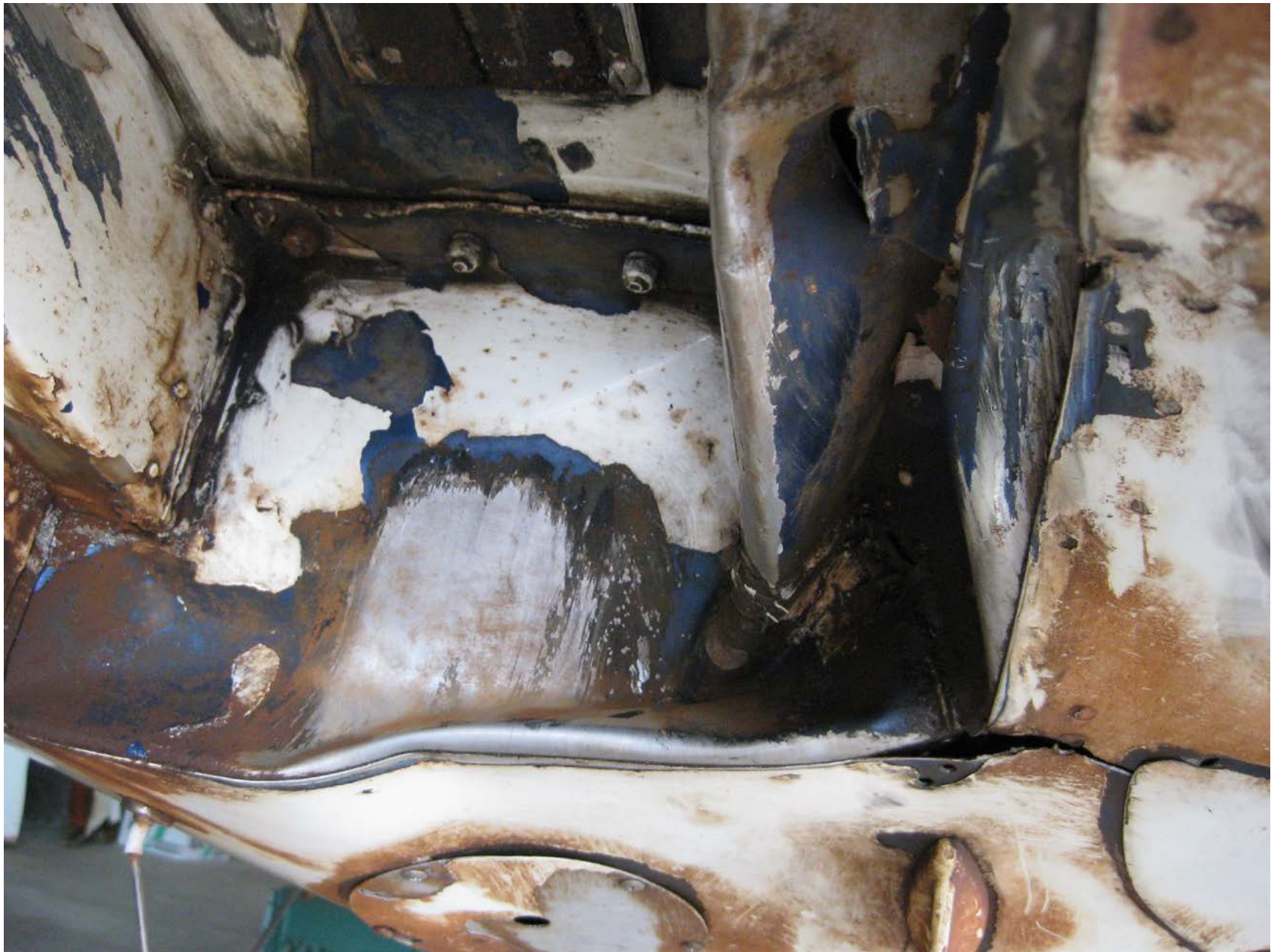
Photo 1 – View of damage to lower fuselage and firewall (Courtesy of FAA)
