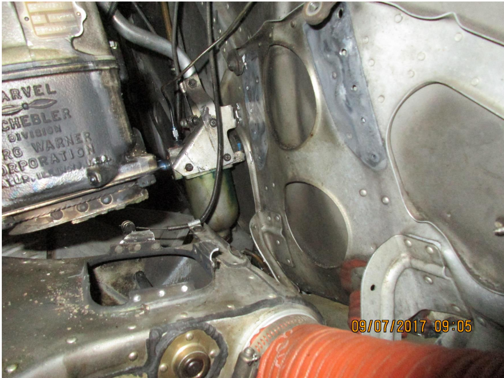
Photo 1 – View of damaged firewall (Photo courtesy of the FAA)
