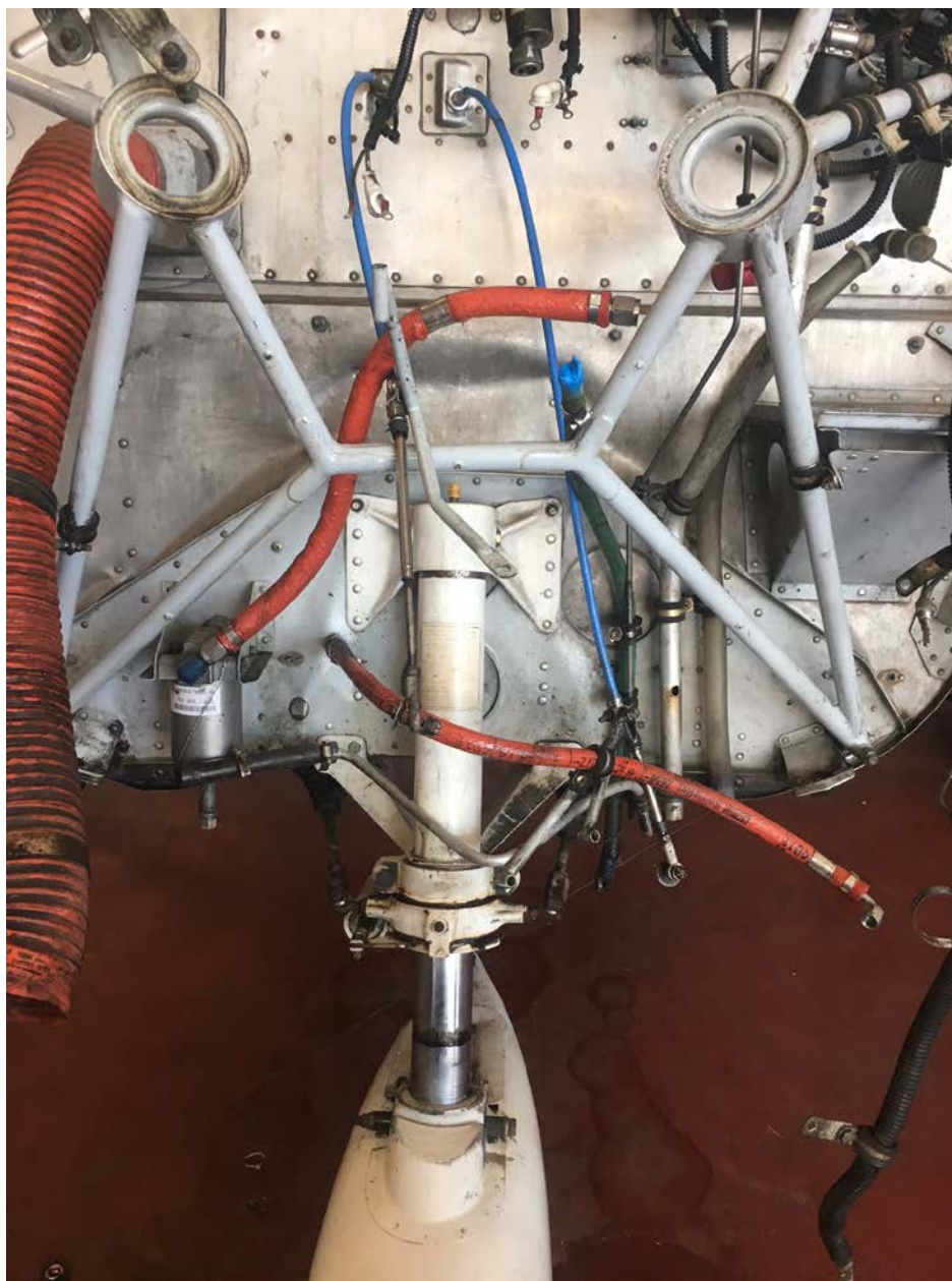
Photo 1 – View of damaged firewall (photo courtesy of the FAA)
