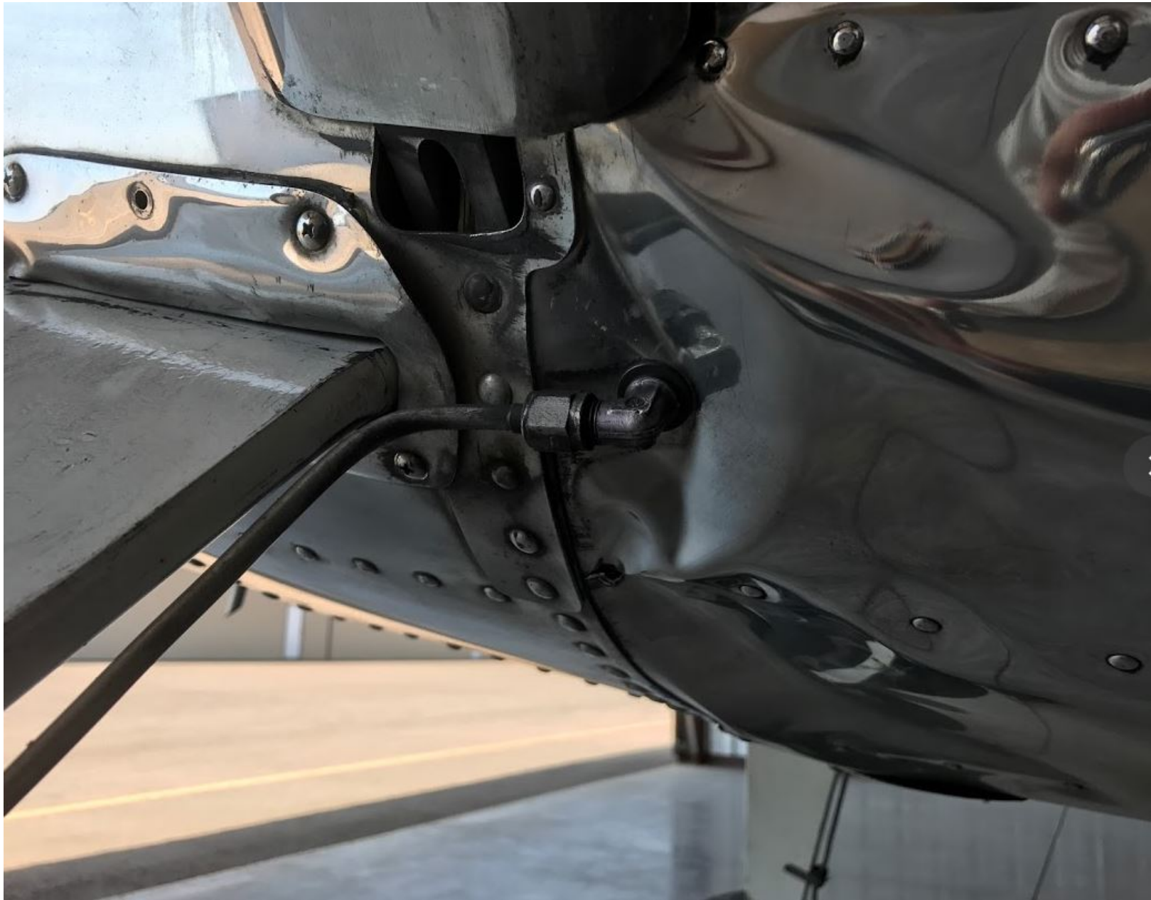
Photo 1 – Substantially Damaged Left Wing Lift Strut (Photo Courtesy of FAA)
