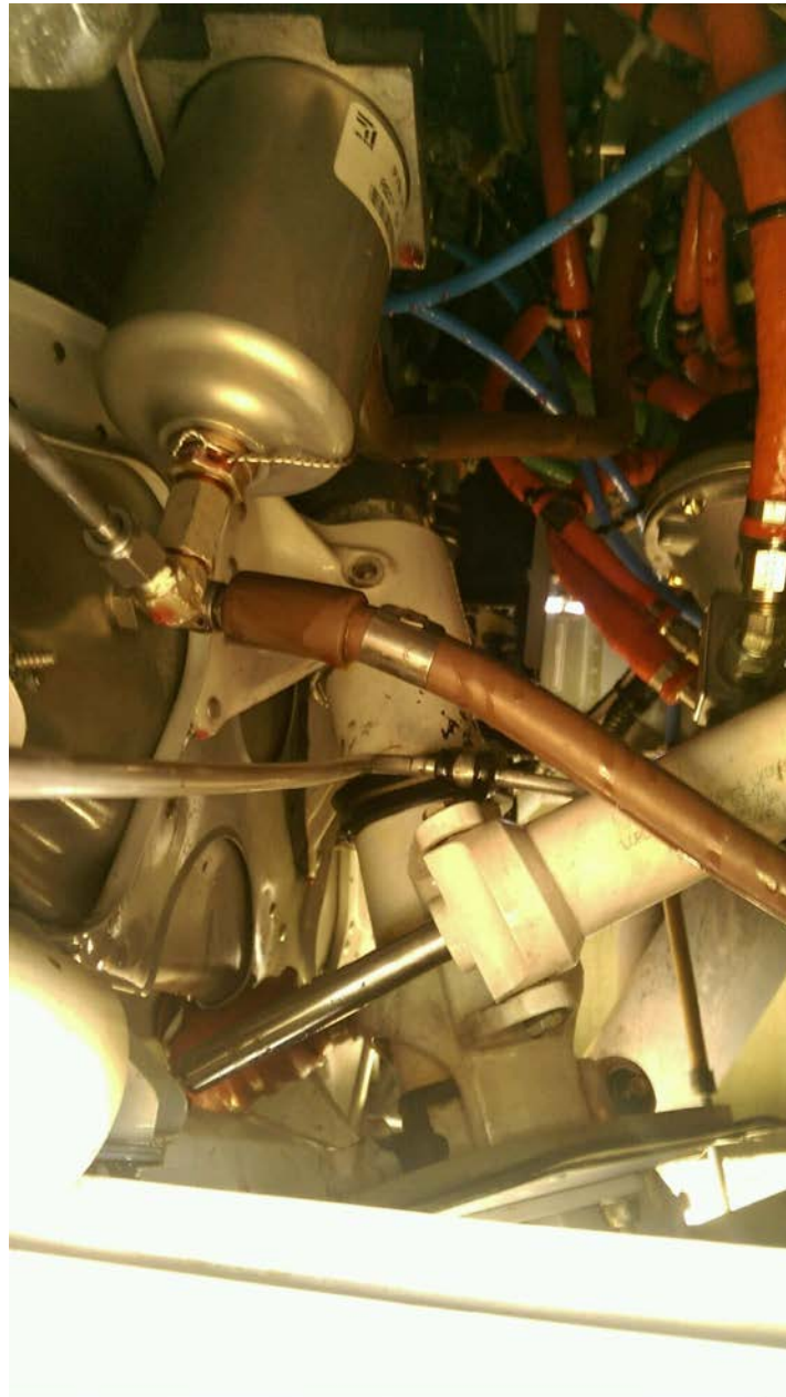
Photo 1 – Substantially Damaged Firewall (Photo Courtesy of FAA)
