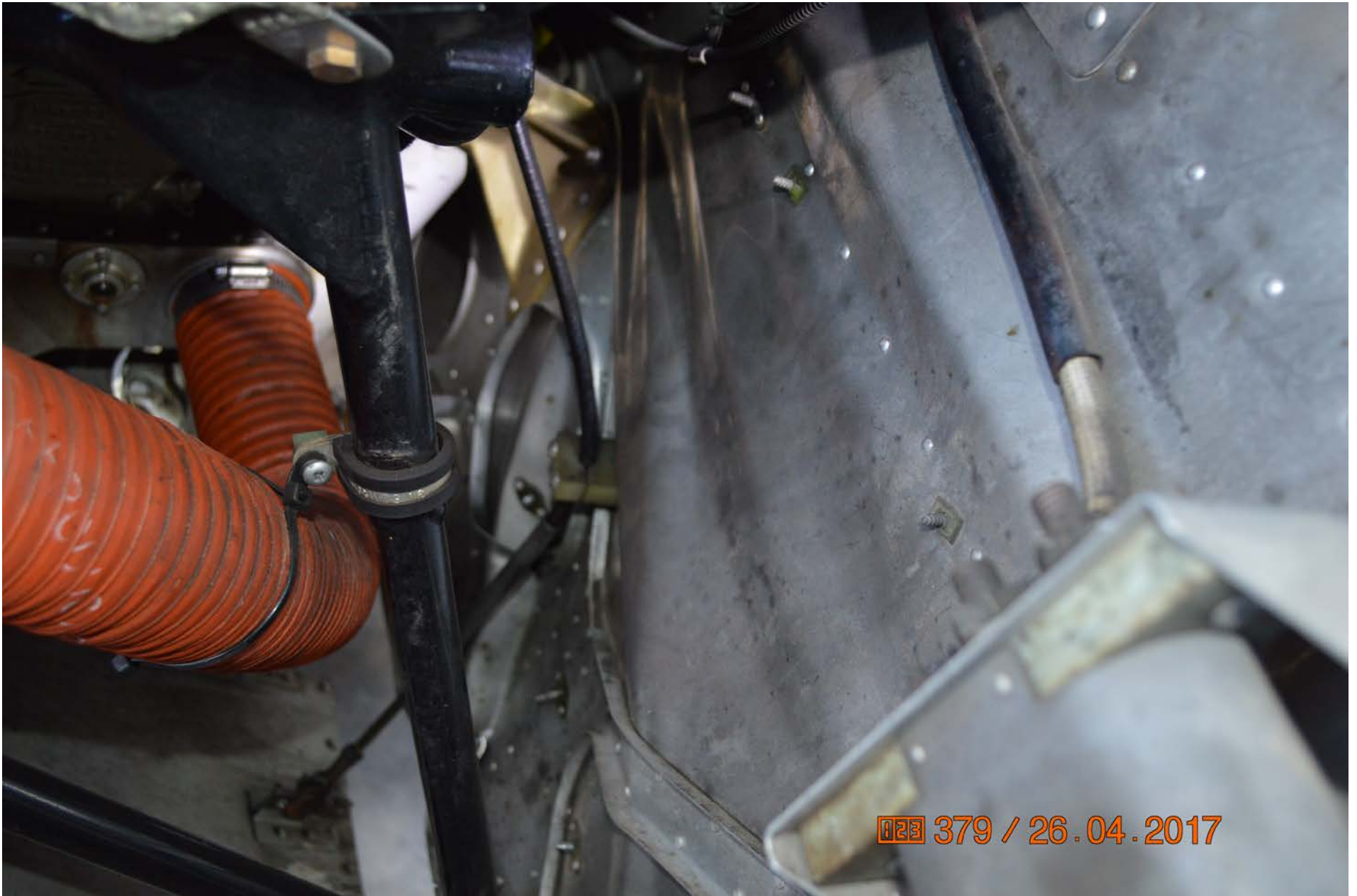
Photo 1 – Substantially Damaged Firewall (Photo Courtesy of FAA)
