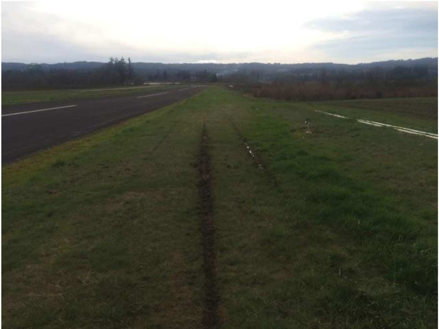
Photo 3 – Tire Tracks Leading Off the Runway (Photo Courtesy of FAA)
