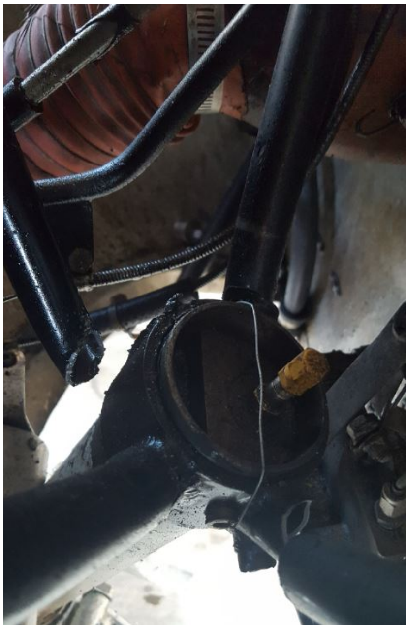
Photo 1 – Damaged Engine Mount (Photo Courtesy of FAA)
