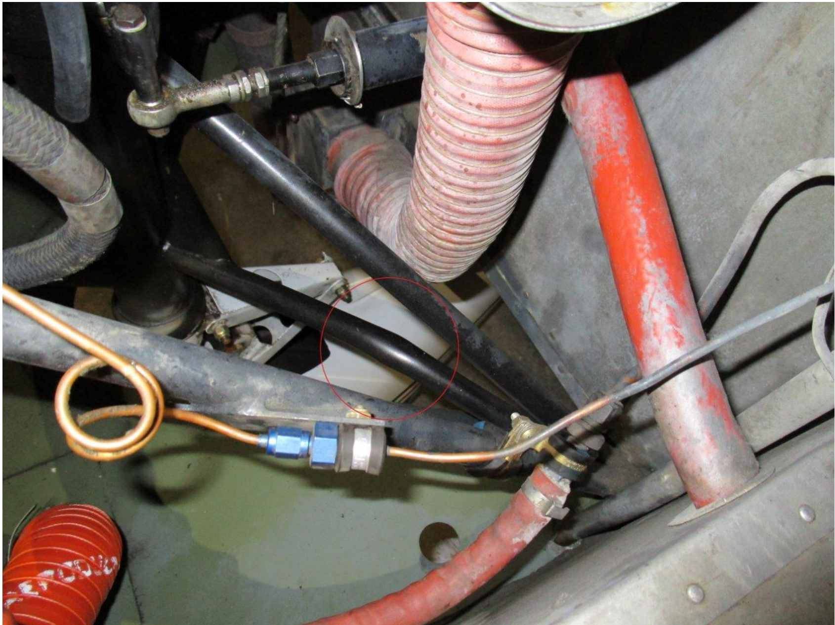
Photo 1 – Damaged Engine Mounts (Photo Courtesy of FAA)
