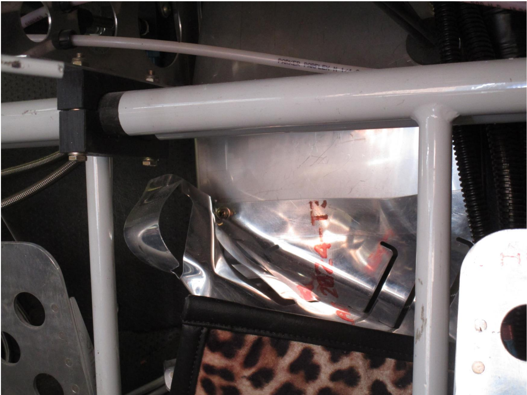
Photo 1 – View of damaged firewall from inside airplane (Photo courtesy of the FAA)
