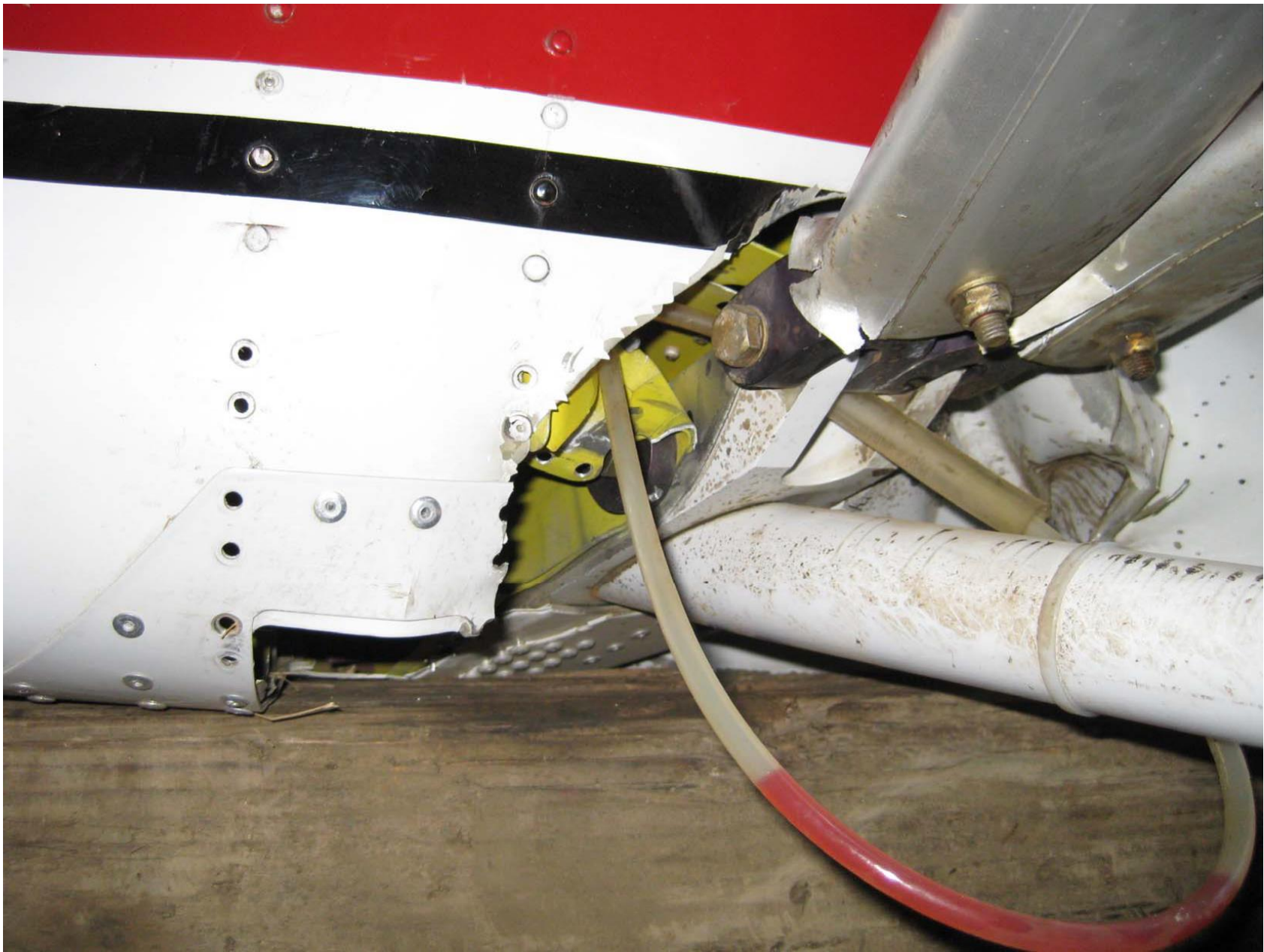
Photo 2 - Bottom view of damaged spar (Photo courtesy of the FAA)
