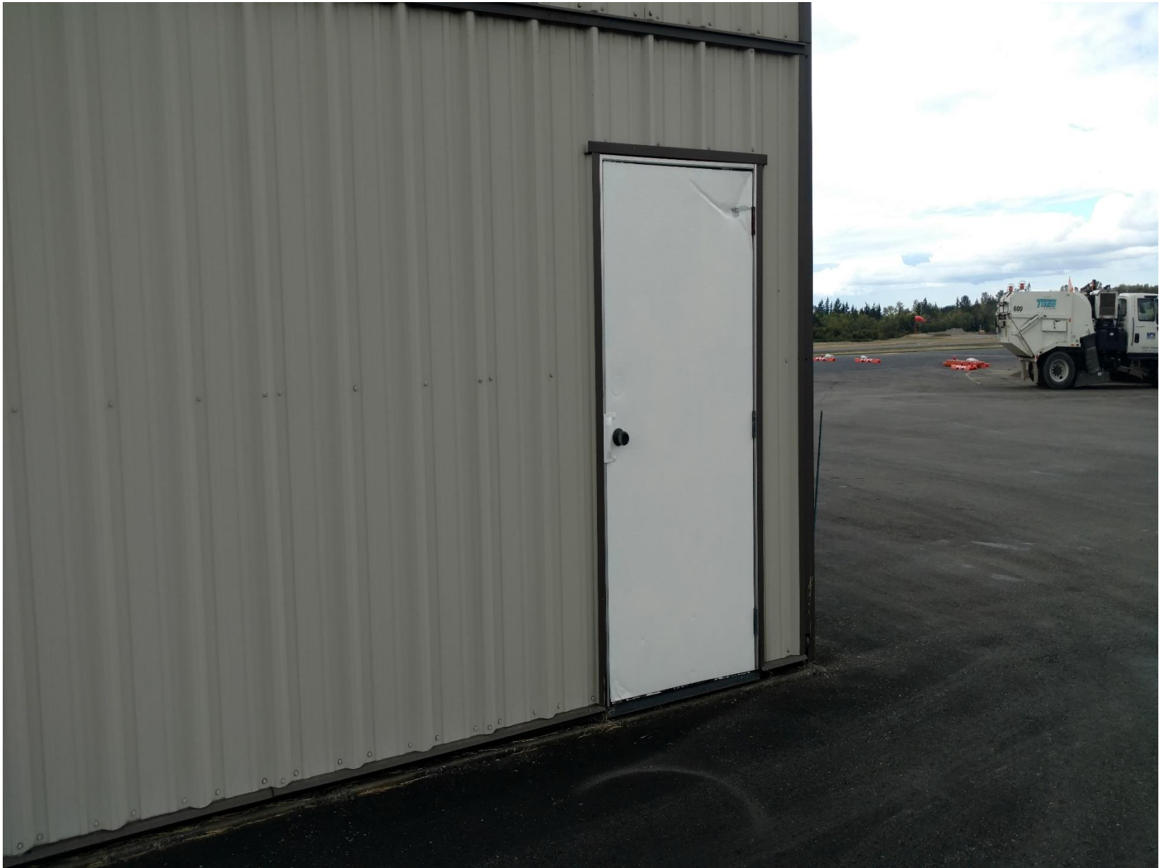
Photo 3 – View of Hangar Door (Courtesy of Pilot)
