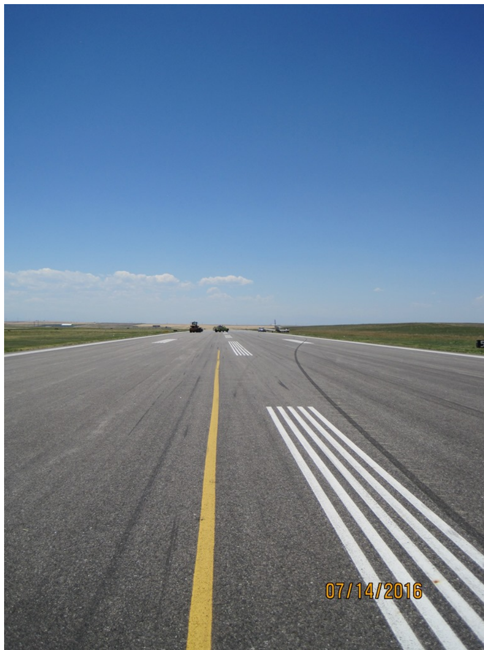
Photo 1 – View of propeller blade strike markings on asphalt (Courtesy of FAA)
