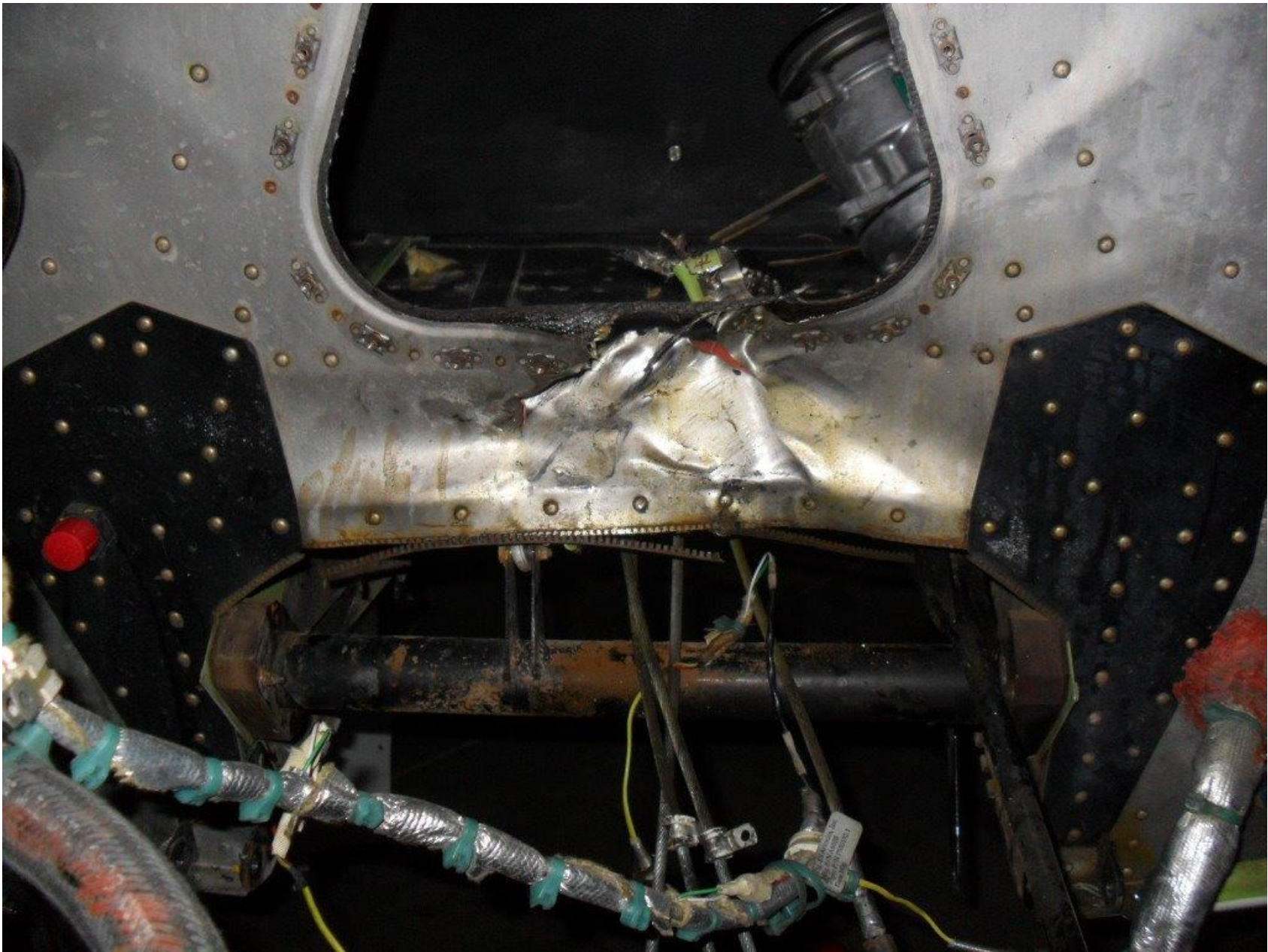
Photo 3 – View of damage to firewall (Courtesy of FAA)
