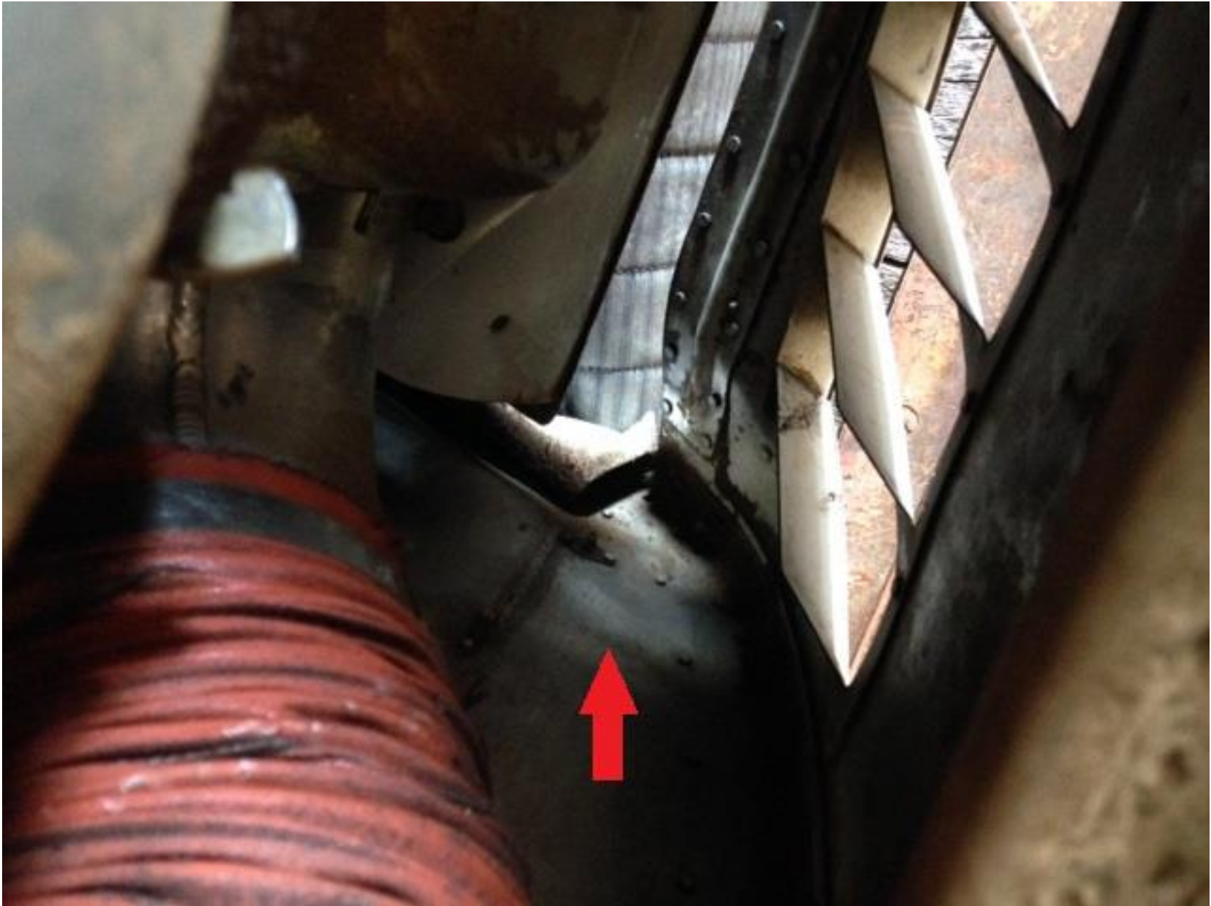
Photo 1 – View of firewall damage from above (photo courtesy of the FAA)
