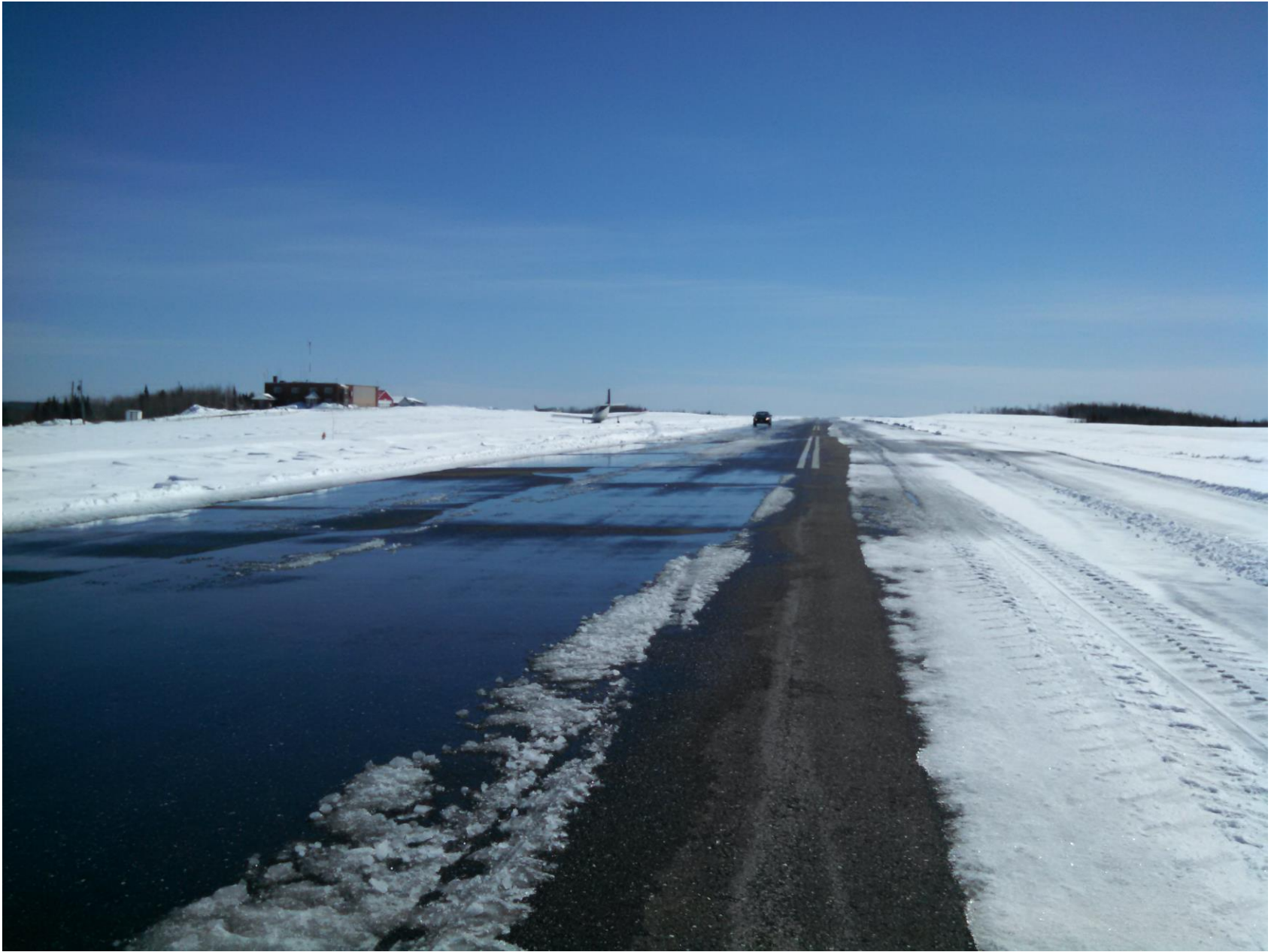
Photo 1 – View of runway (courtesy of the FAA)
