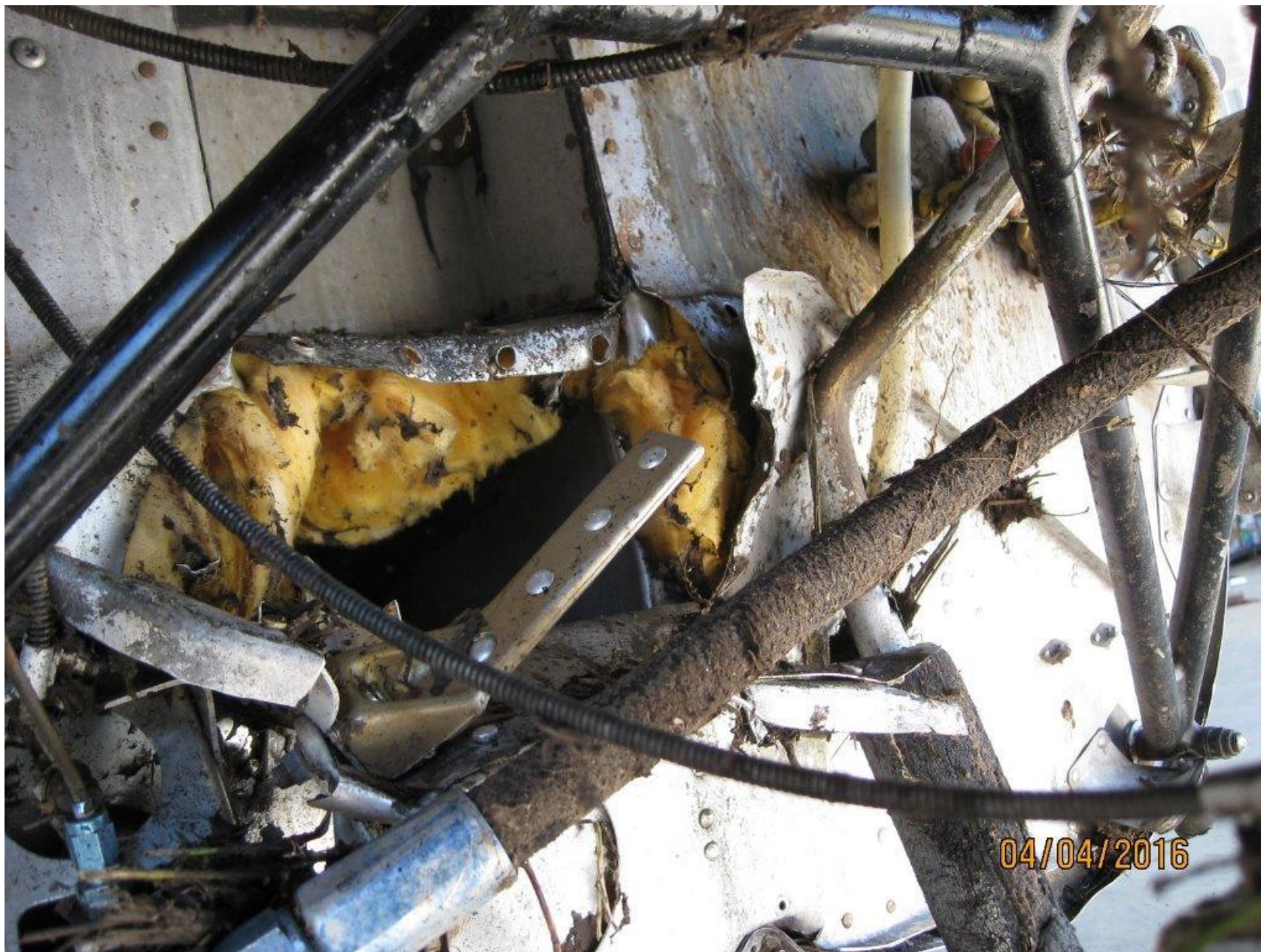
Photo 2 – View of firewall (courtesy of the FAA)
