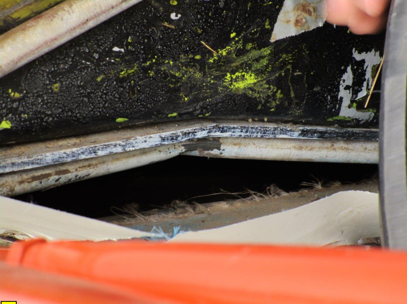
Photo 2 – Damage to Firewall (Courtesy of FAA)
