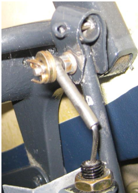
FAA provided photograph showing two washers and nut installed on pin.
