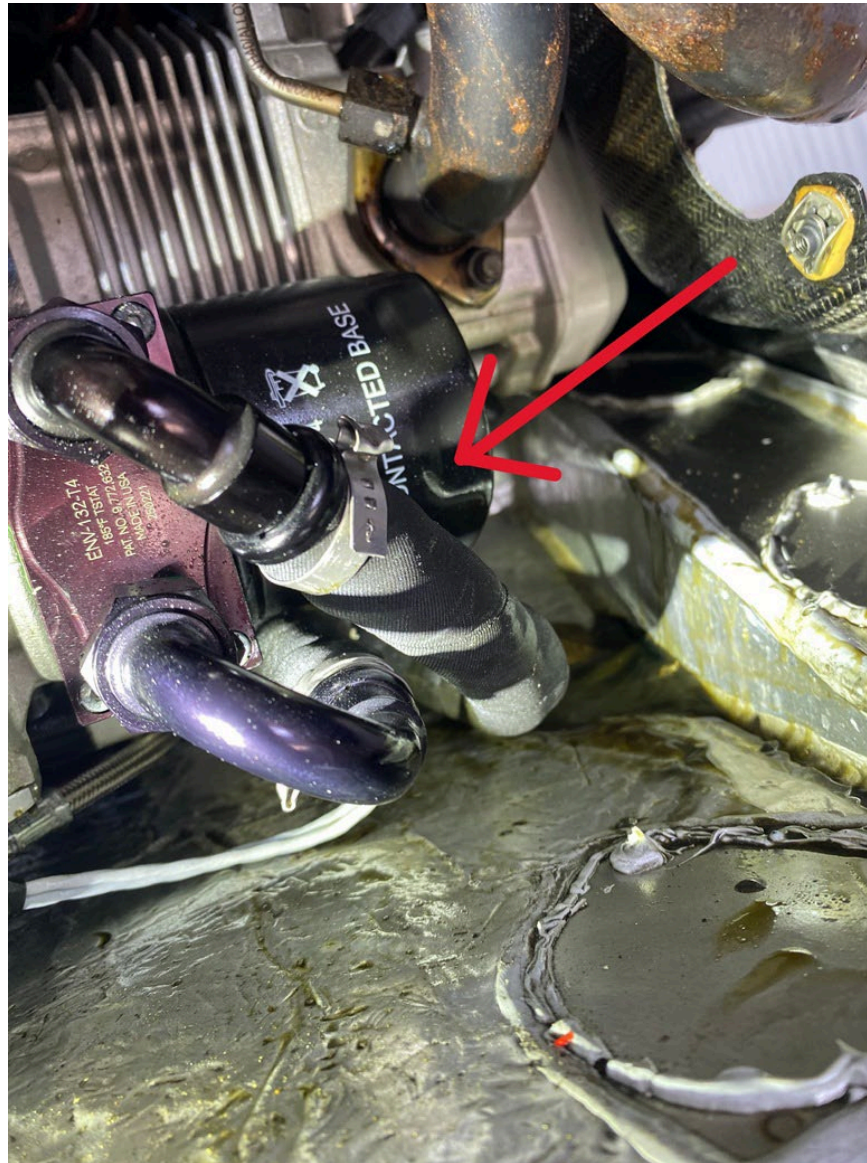
Photograph 3 - Oil Line Attached With Clamp at Oil Pump Fitting (Courtesy of FAA)
