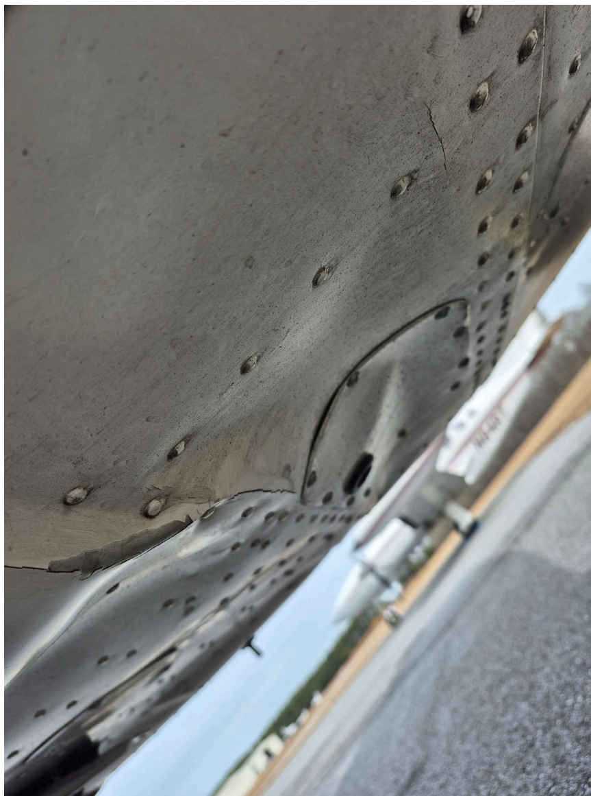
Photograph 2 - View of the Bottom Fuselage Showing Structural Buckling Damage near Fuselage Station 17 (Courtesy of FAA)
