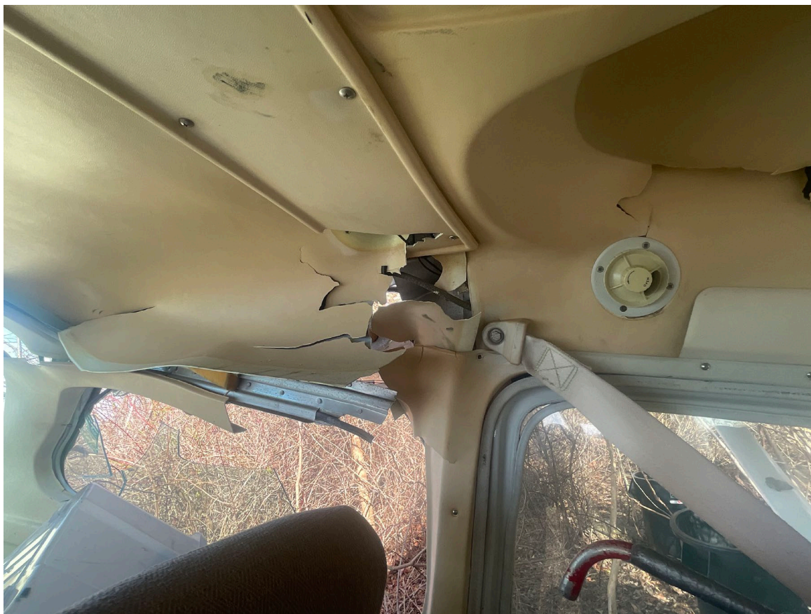
Photograph 4 - Interior Paneling and Fuselage Damage (Courtesy of FAA)
