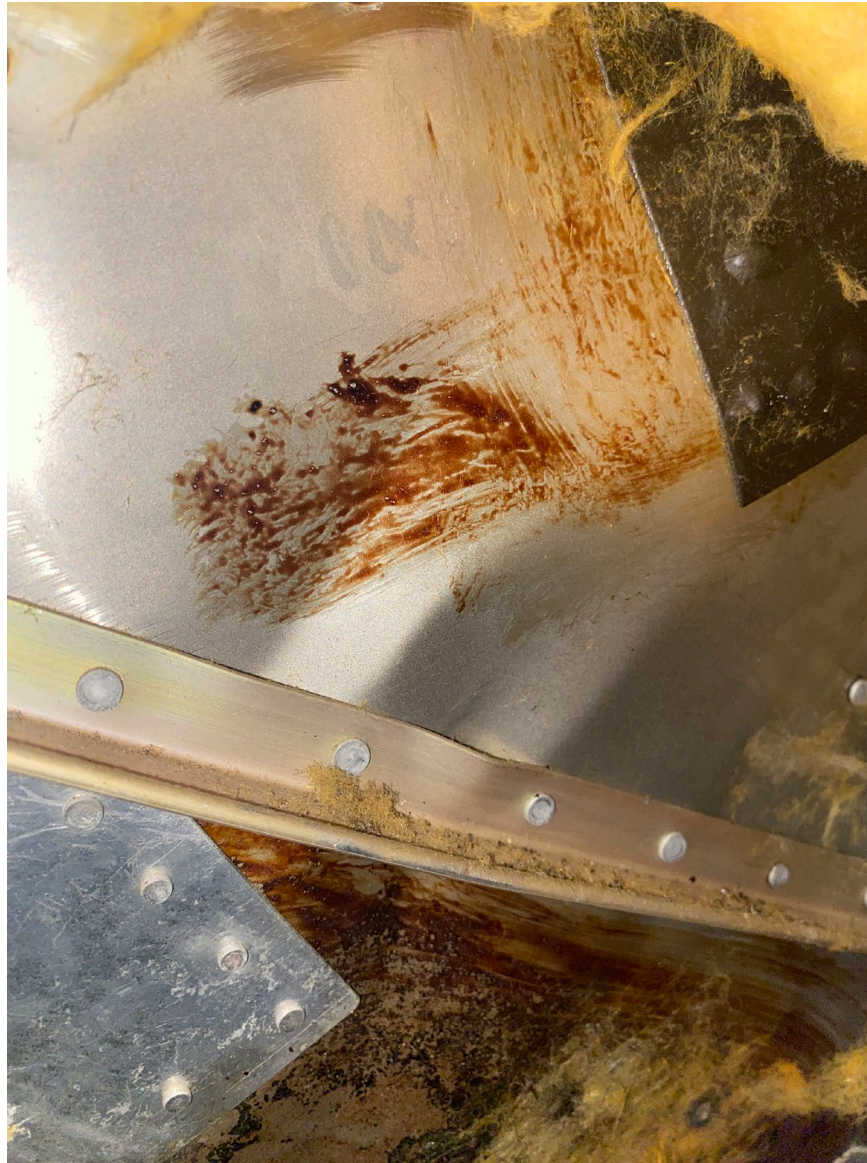
Photograph 3 - Damaged Cockpit-Side Firewall Stiffener (Courtesy of FAA)
