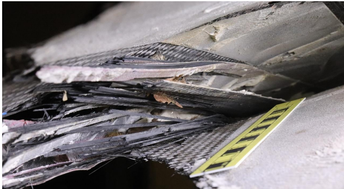
Figure 19. Images of upper and lower spars splintering about 26 inches outboard of the doublers.
