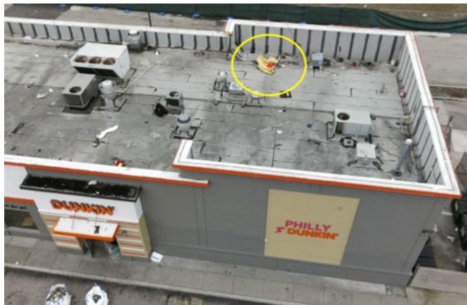
Figure 22: Aerial view of the aircraft's life raft on the roof of the Dunkin', 1230 Cottman Avenue, Philadelphia, PA, looking north. (February 2, 2025, annotation by NTSB).
