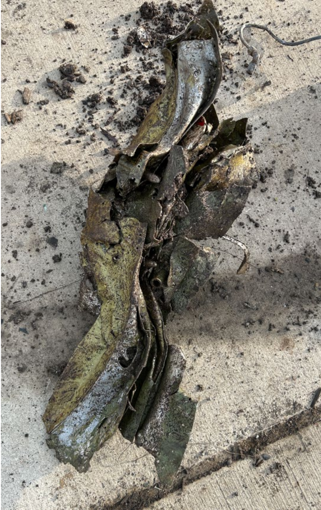
Figure 37: Main Entry Door Frame
