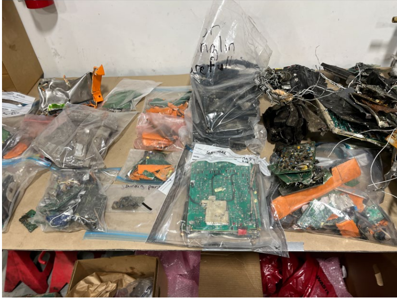
Figure 53: Circuit Breaker Panels and Miscellaneous Electronic Equipment
