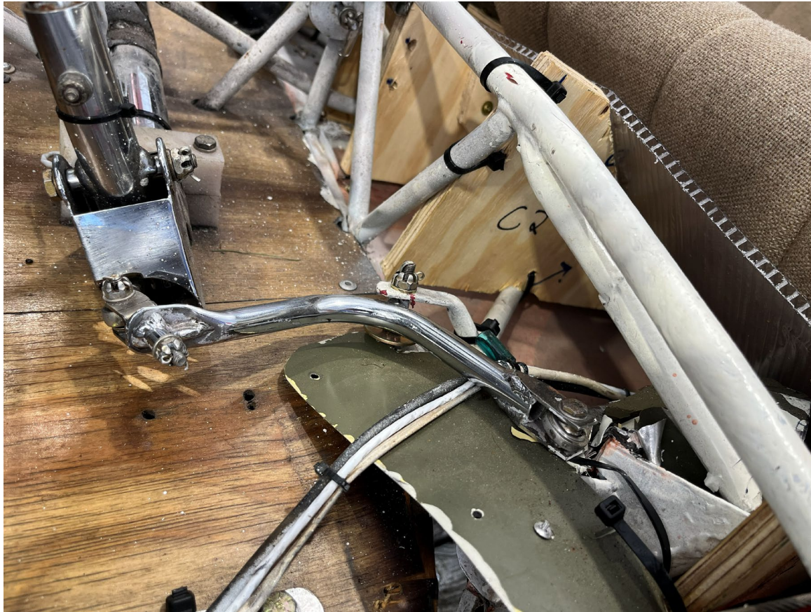
Photograph 3 - Left Forward Landing Gear Strut Punched Through Cockpit Floor (Courtesy of FAA)
