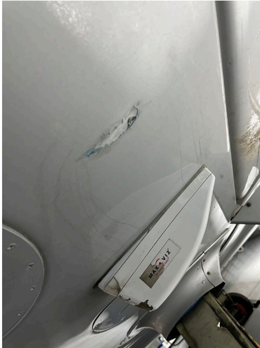
Photograph 3 - Left Fuel Cell Breach (Courtesy of FAA)
