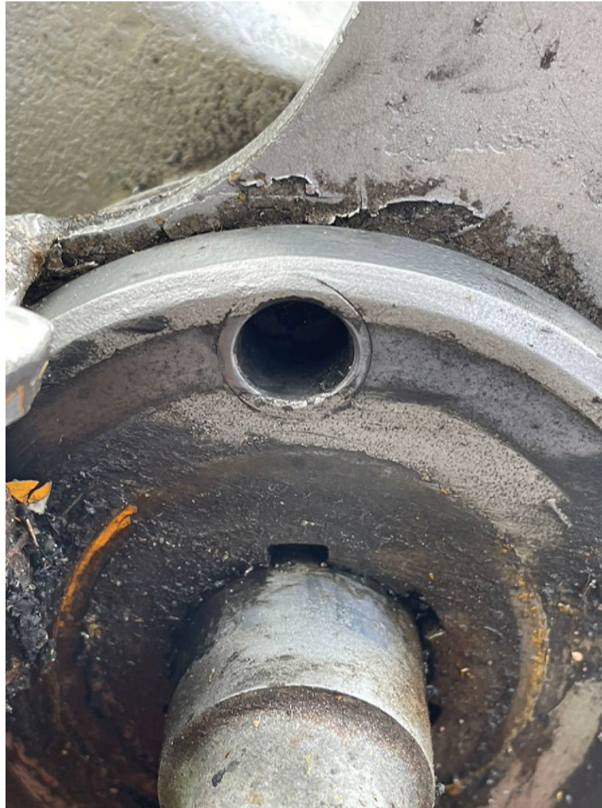
Photograph 7 - Wear to locking pin engagement hole (Courtesy of FAA)
