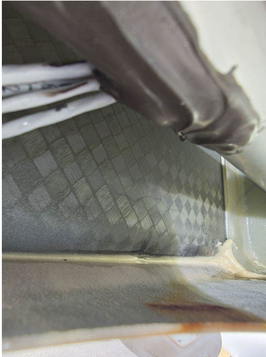
Photograph 3 - Wing Spar Crack (Courtesy of FAA)
