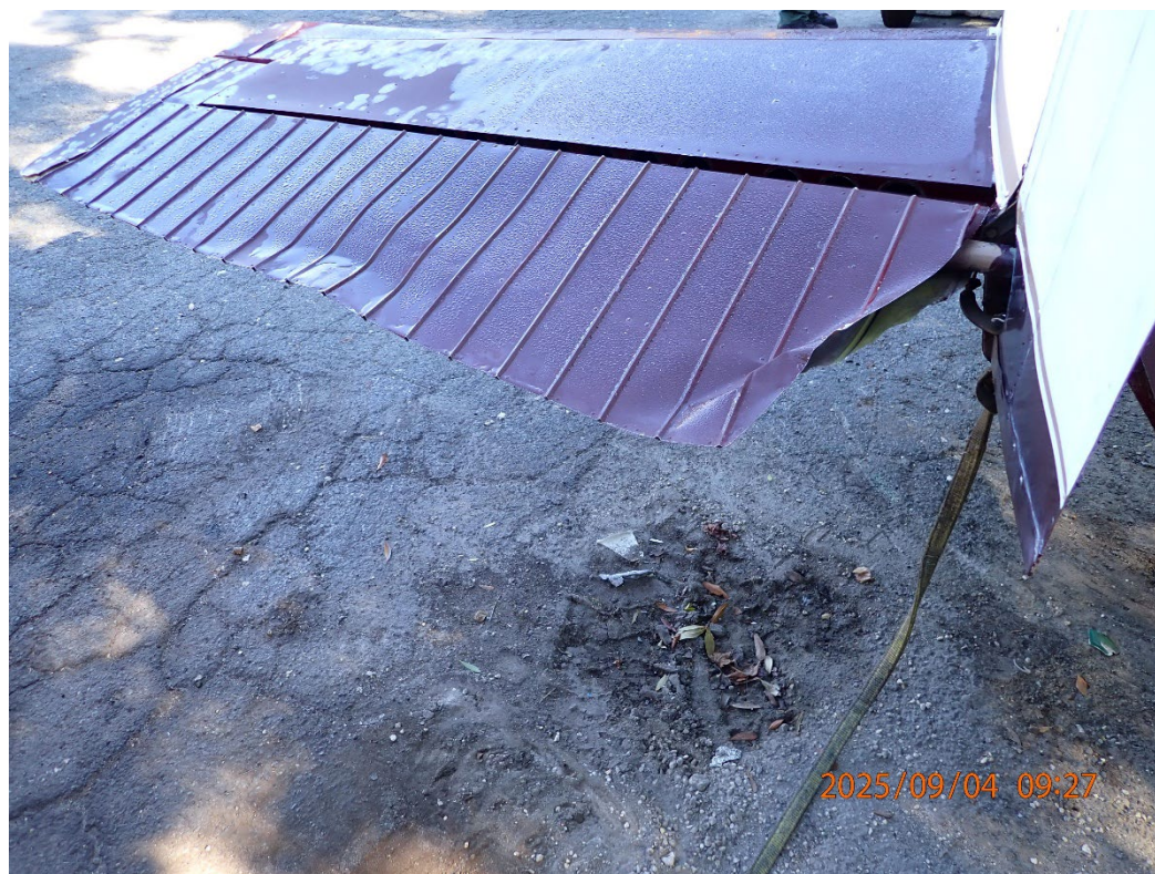
Photo 5: View of damage to the left elevator.
