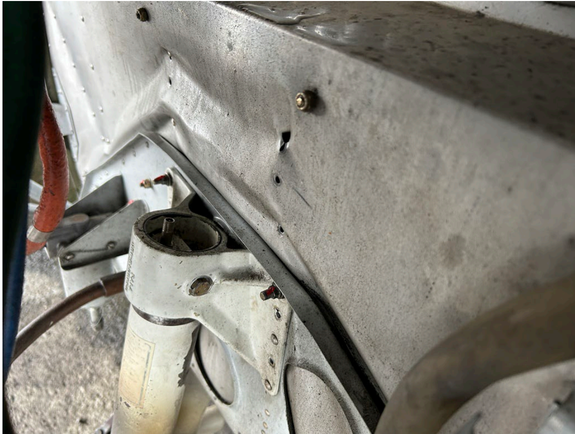
Photograph 2 - Firewall Damage (Courtesy of FAA)
