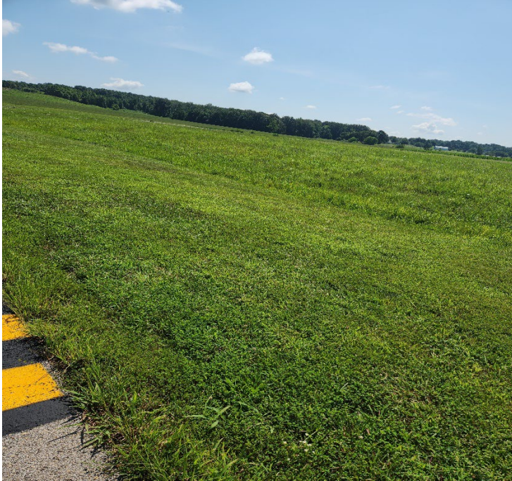
Turn around area - Heading towards runway 6 View #2
