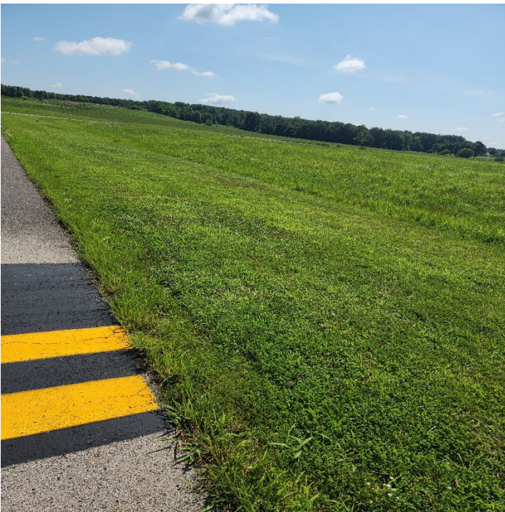
Turn around area - Heading towards runway 6 View #3
