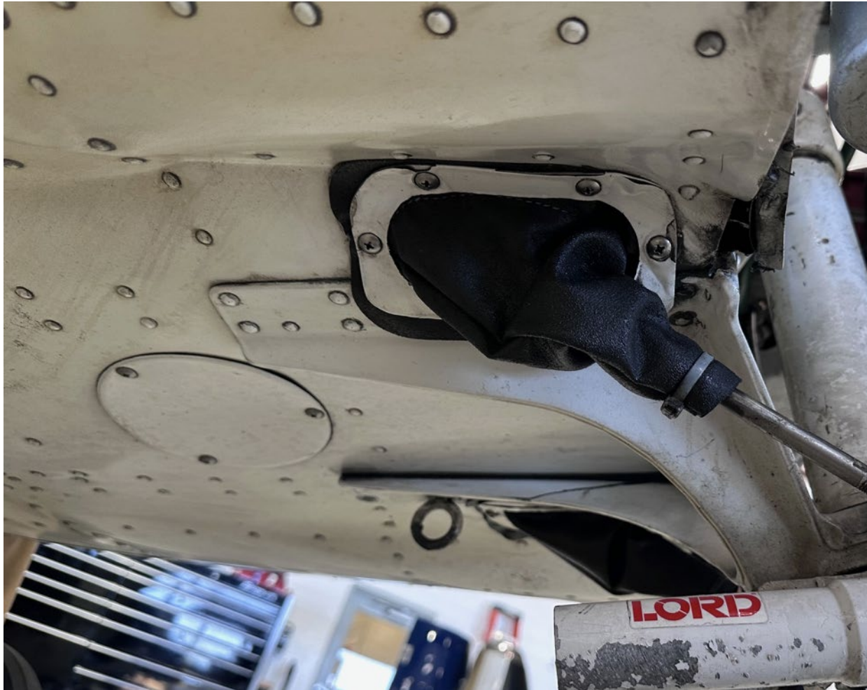
Photograph 7 - Close Up of Firewall Tunnel Juncture (Courtesy of American Aviation)
