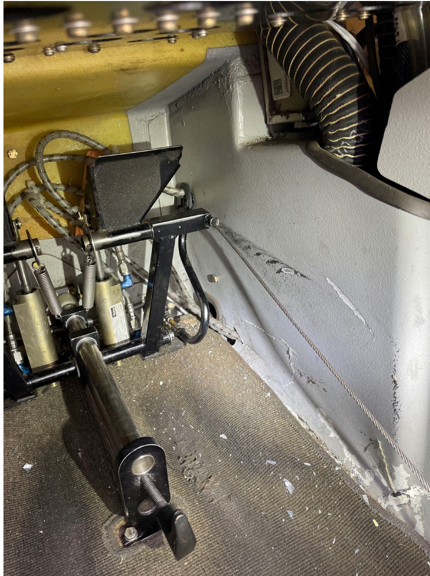
Photograph 2 - Pedestal structure accident damage (Courtesy of FAA)
