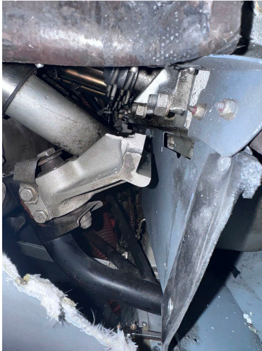
Photograph 3 - Broken Airplane Engine Mount (Courtesy of C. Blas)
