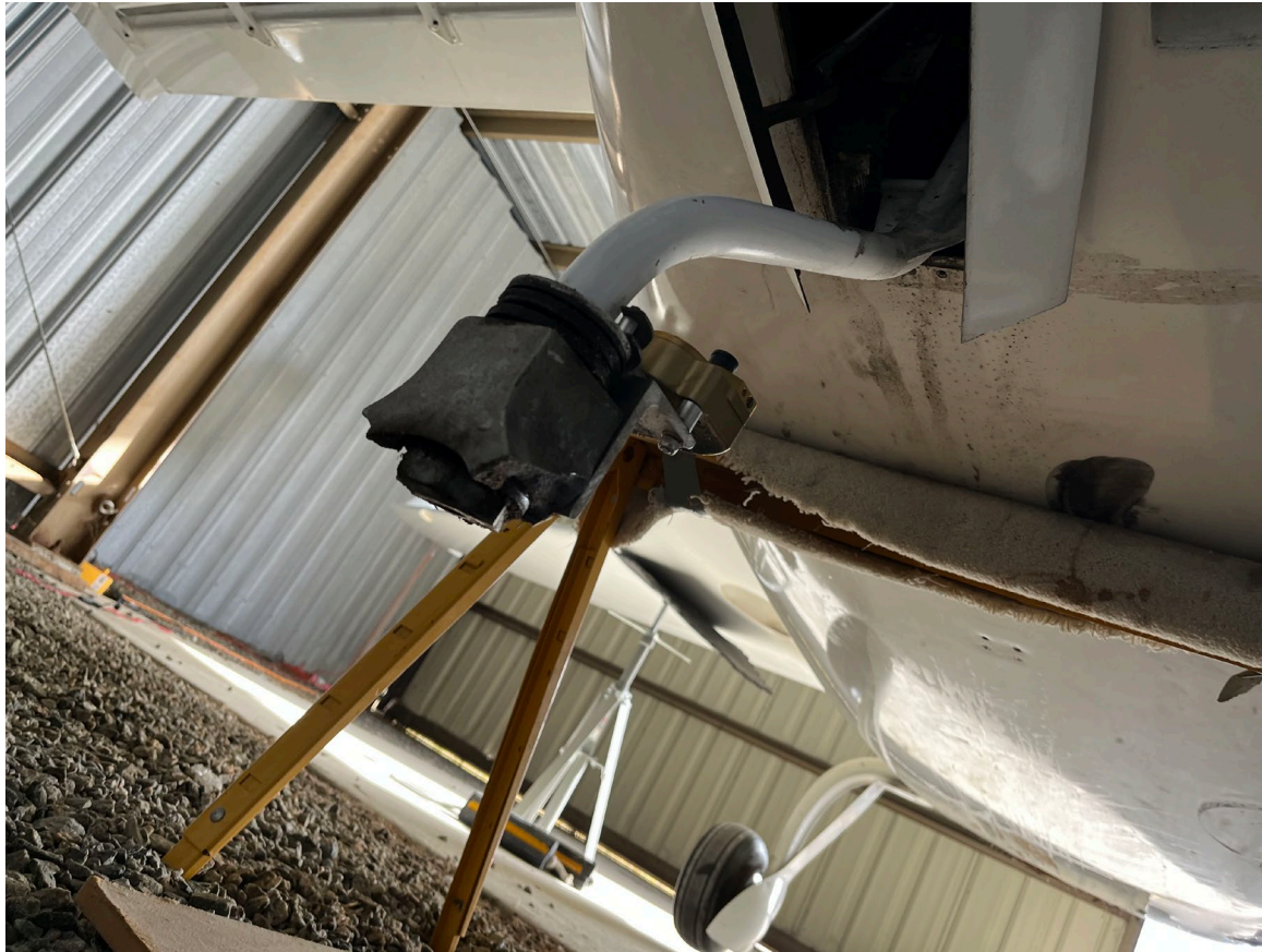
Photograph 2 - Nose landing gear damage (Courtesy of FAA)
