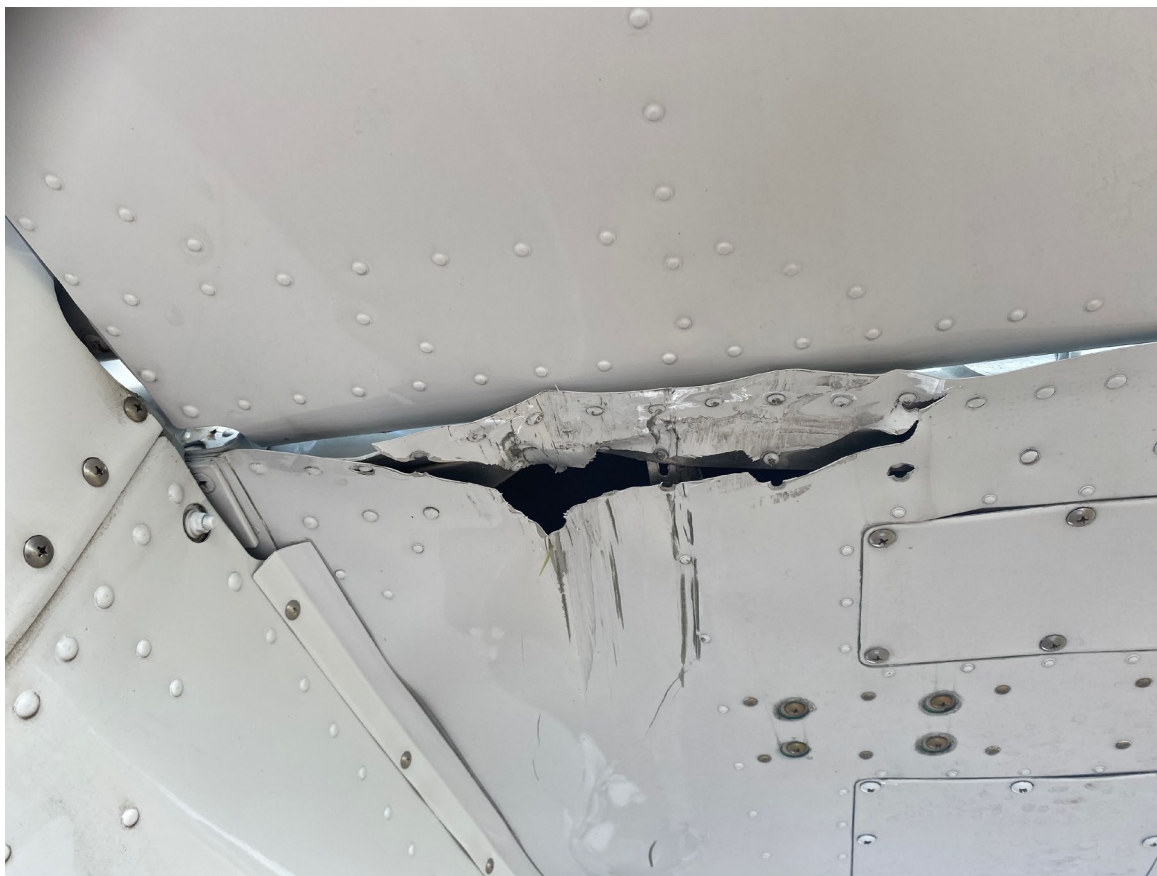
Photograph 4 - bottom right horizontal stabilizer accident damage (Courtesy of airplane owner)
