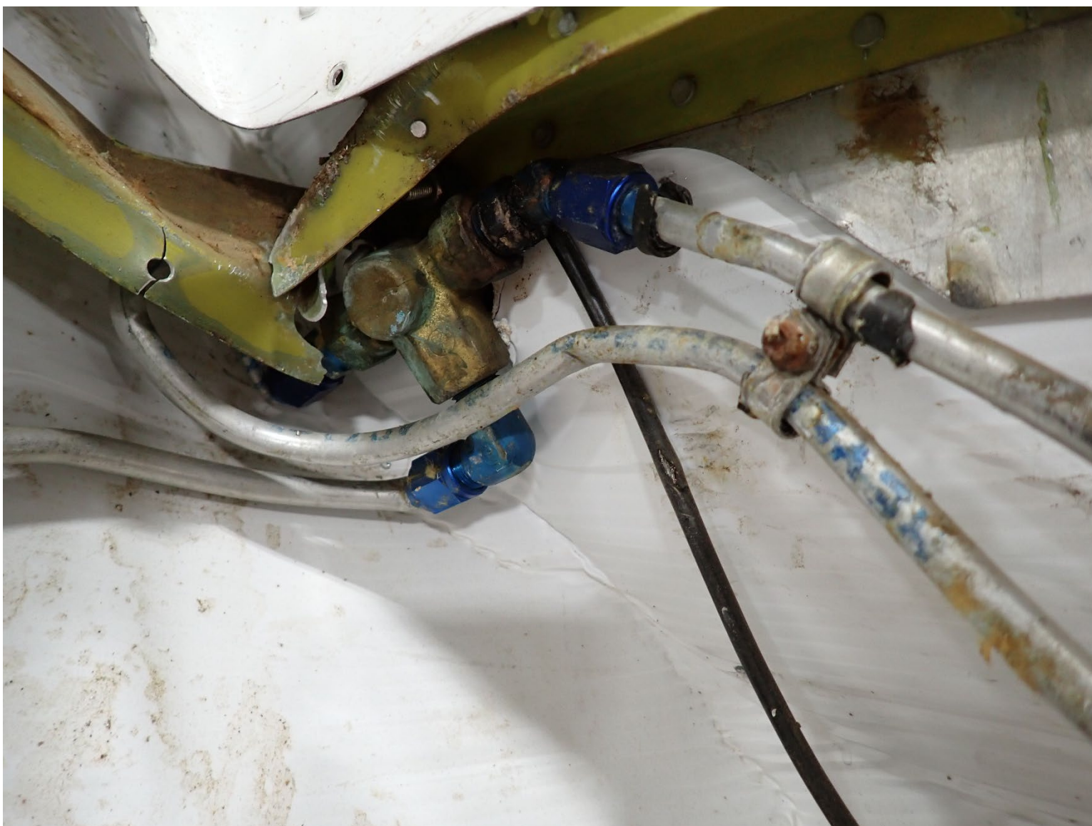
Photograph 9 - Fuel selector valve
