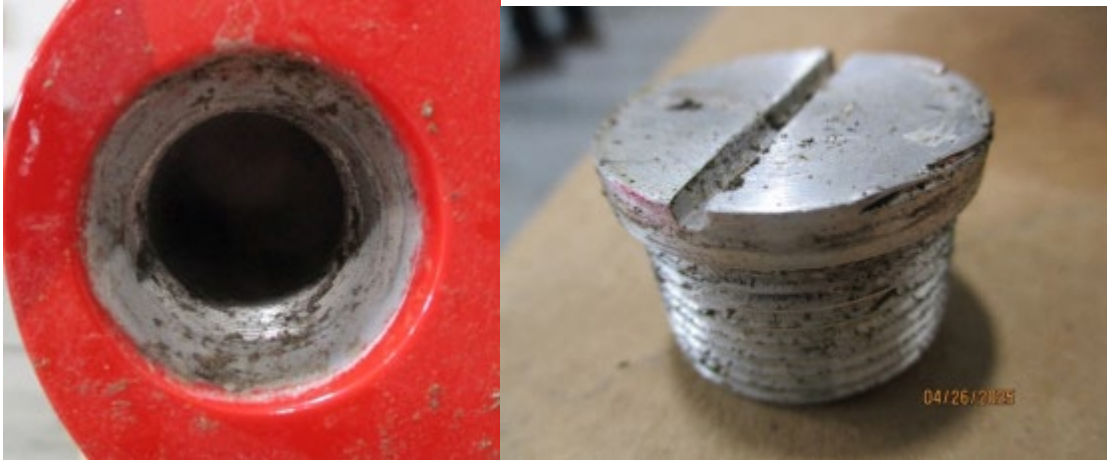
Figure. Left elevator counterweight installation hole (left) and recovered counterweight plug (right). Gouging and paint transfer are visible on the counterweight plug.
