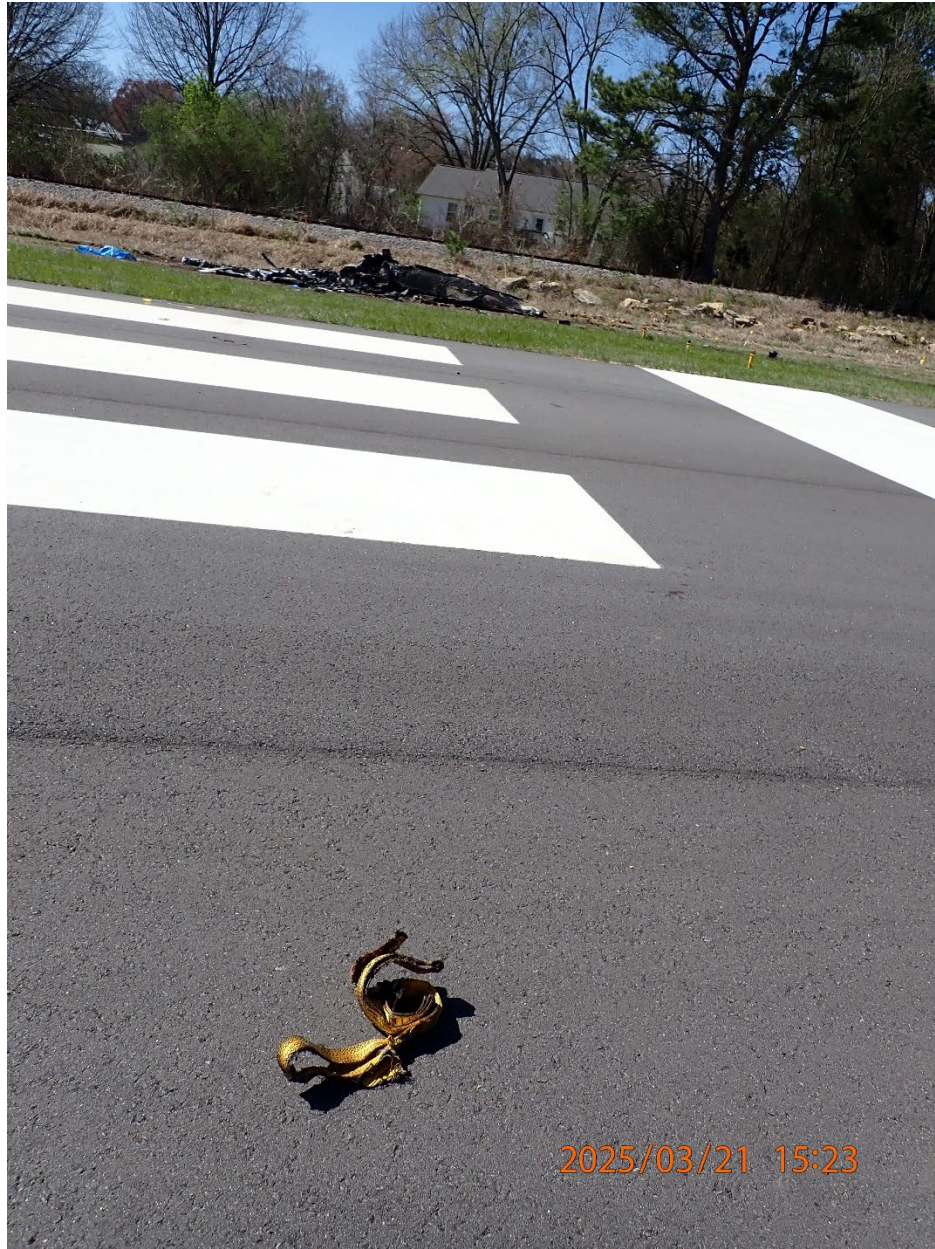
Photo 13: View of a portion of a CAPS strap on the runway.
