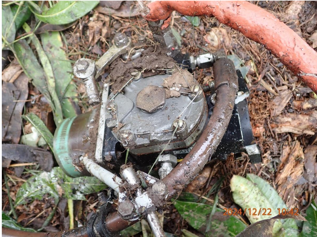
Photo 36: View of the fuel injector assembly.
