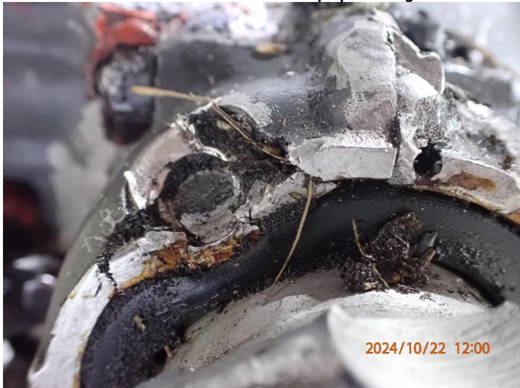
Photo 32: Impact damage at the flange of the crankshaft.
